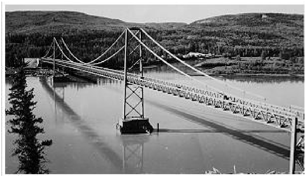
The suspension bridge over the Peace River near Taylor BC (1942 to 1952)
