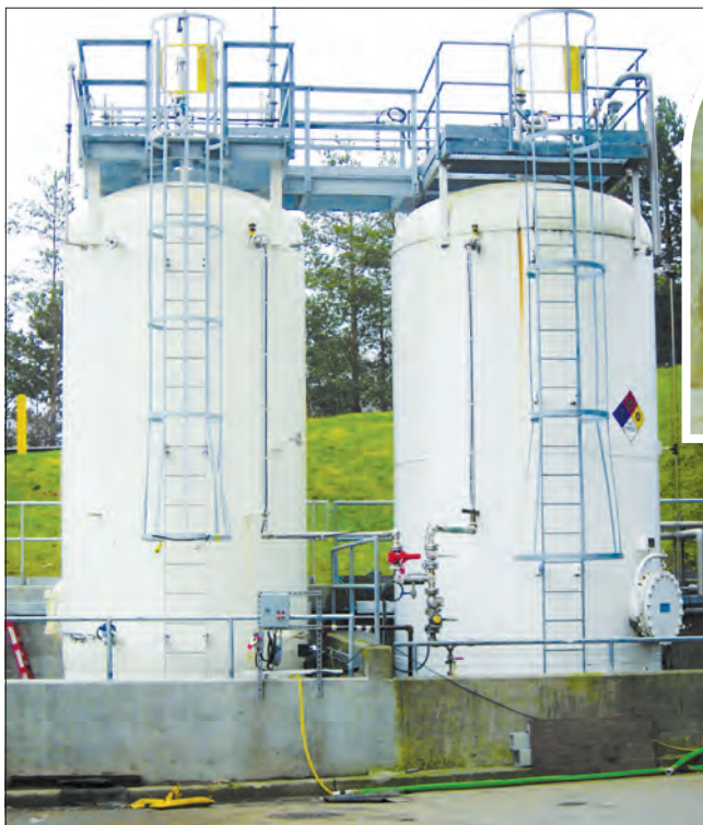
LEFT: Addition of a second ammonia storage tank increases ammonia storage and supply.
